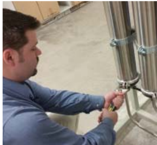
Reverse Osmosis Systems
